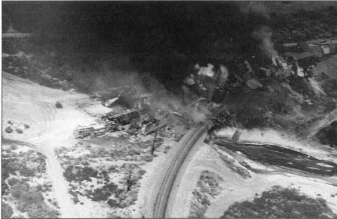
Figure 4.--Accident scene, looking northwest
